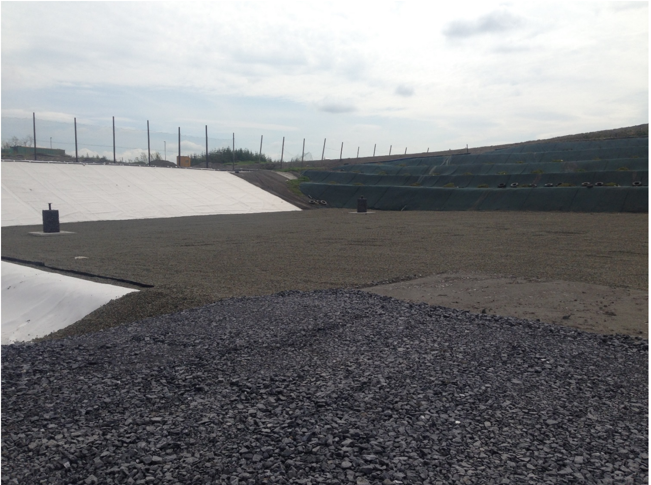
Plate 2-3: Lined cells at Knockharley Landfill
