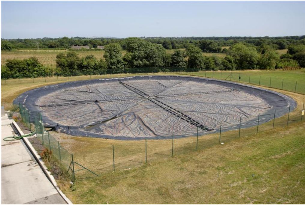
Plate 2-4: Covered Leachate Lagoon
